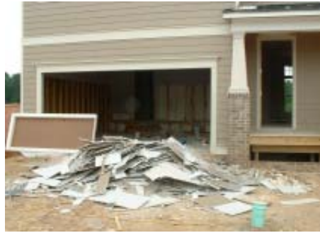
Unground wallboard awaits grinding and land-applying at a new construction site.
